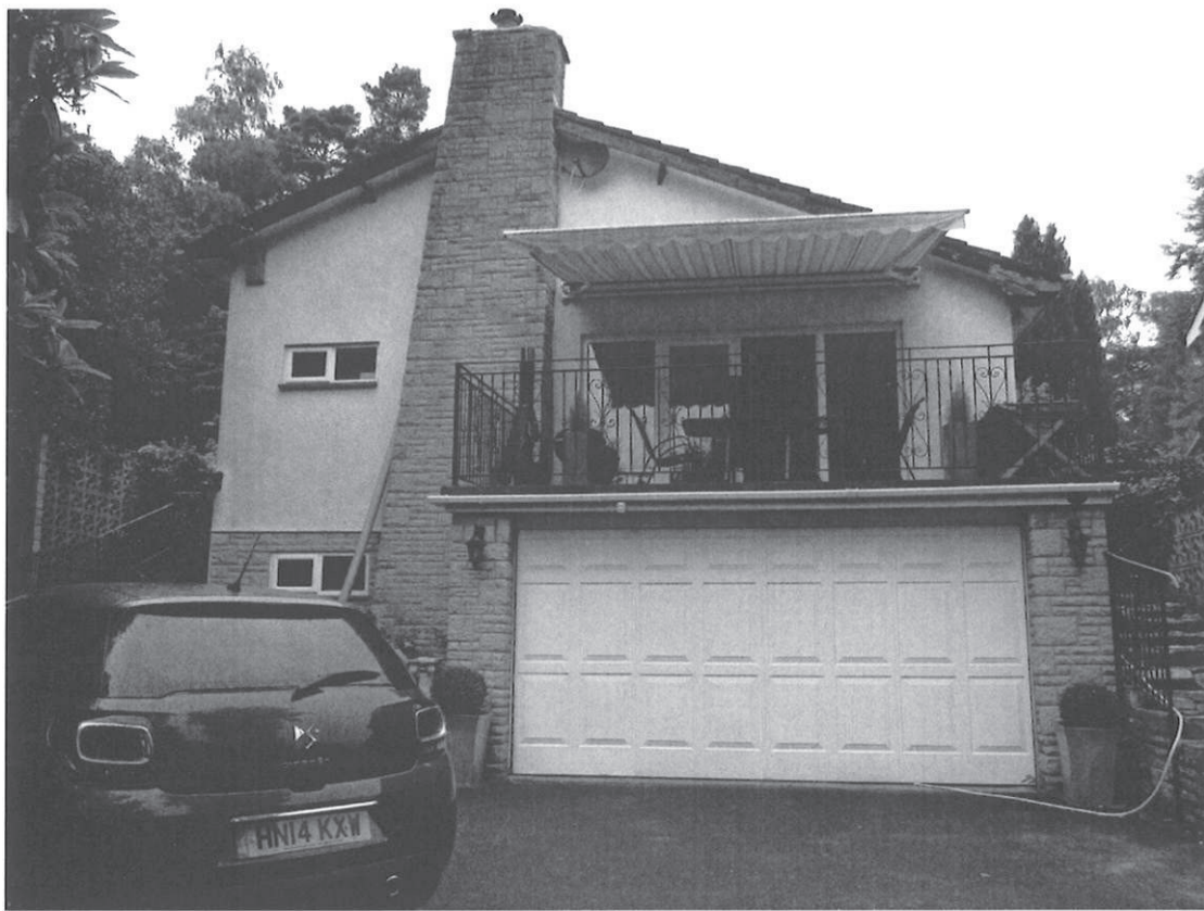
Application site – Rear Elevation
